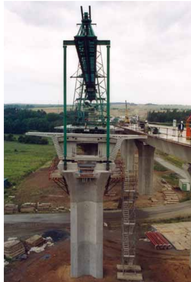
Uhlavu Bridge, Pilsen, Czech Republic
