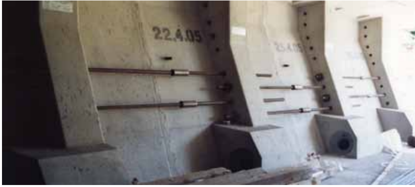
Typical Coupling, Uhlavu Bridge, Pilsen, Czech Republic
