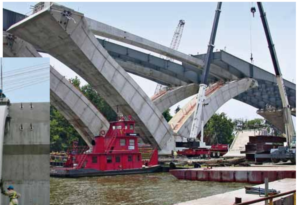
Woodrow Wilson Bridge, Washington, D.C., USA
