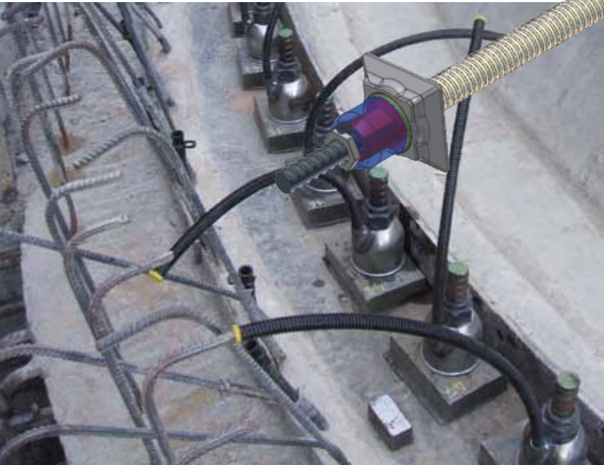
Bonded bar tendon, design QR-plate, square and rectangular solid plates
