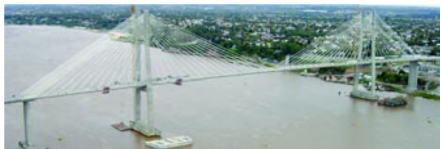
Rosario Victoria Bridge, Argentina
