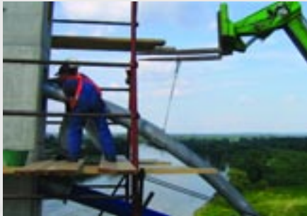
Saddle Pipe Installation
