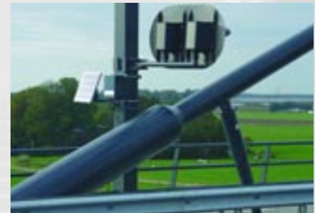
Installed External Damper
