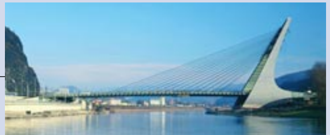
Ústí nad Labem Bridge, Czech. Republic 30 DYNA Bond® Stay Cables Maximum cable length: 143 m Cable sizes: DB-P12, DB-P19
