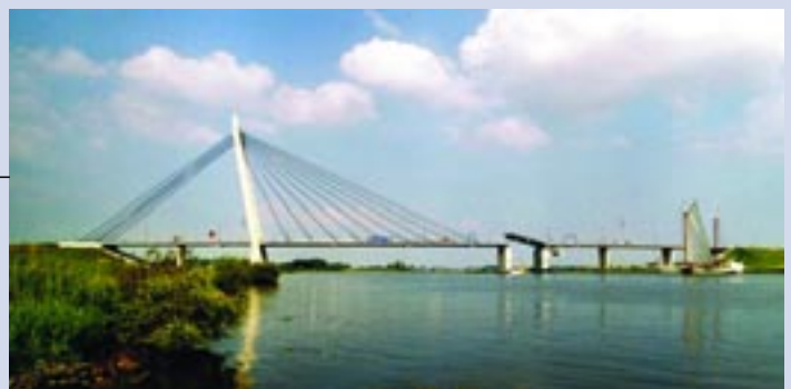
Kampen Bridge, Netherlands 24 DYNA Grip® Stay Cables Maximum cable length: 163 m Cable sizes: DG-P37, DG-P55, DG-P91
