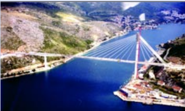
Dubrovnik Bridge, Croatia 38 DYNA Bond® Stay Cables Maximum cable length: 223 m Cable sizes: DB-P27, DB-P61
