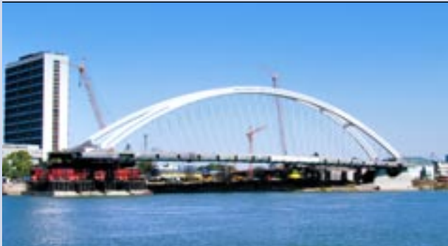
Apollo-Bridge, Slovakia 66 DYNA Grip® Stay Cables Maximum cable length: 37 m Cable size: DG-P12
