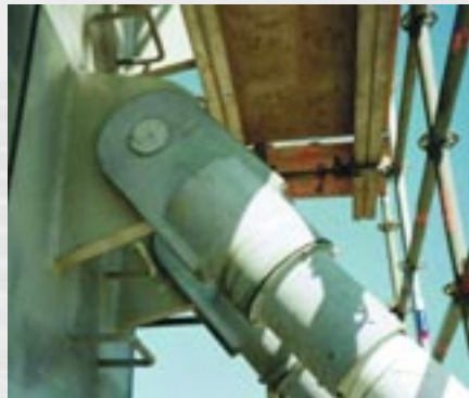
Clevis Anchorage
