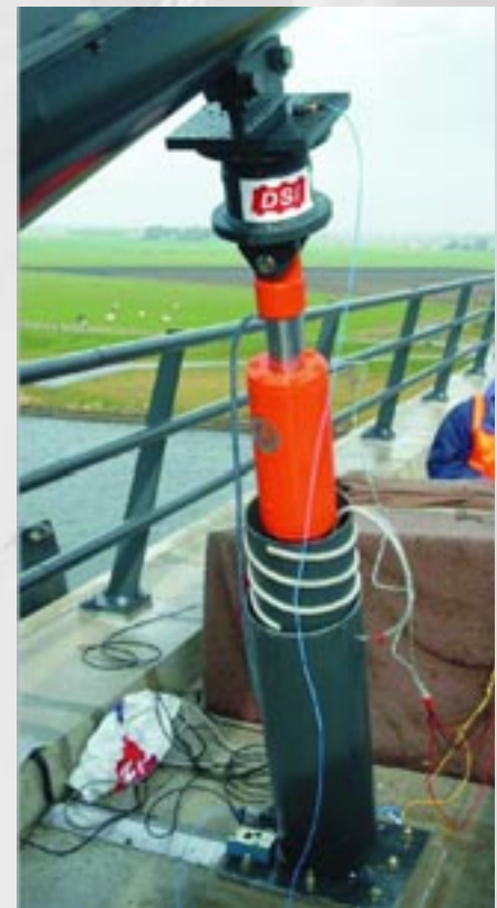
Test Installation of a Hydraulic Damper
