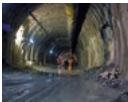
Metsovo Tunnel, Metsovo, Greece
