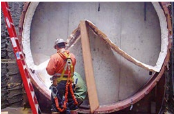
Fixation of the BULLFLEX® o-ring sealing in the lower area
