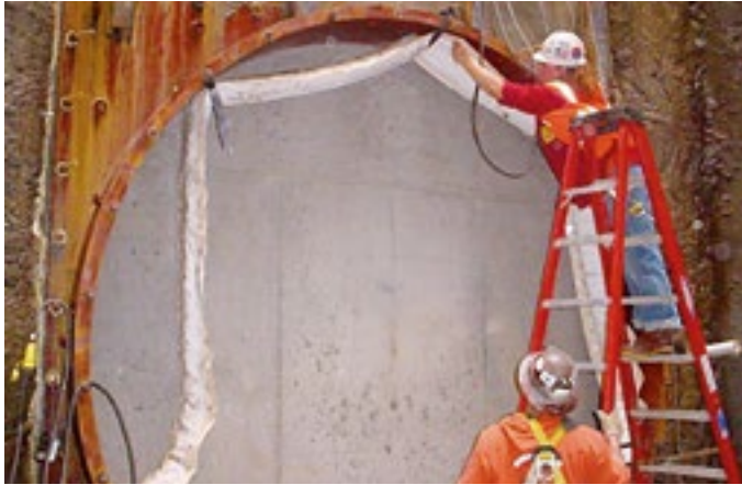
Mounting of the BULLFLEX® o-ring sealing for marking of the welding spots
