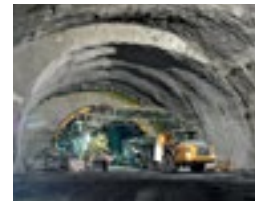
Sentvid Tunnel, Ljubljana, Slovenia
