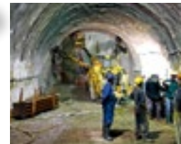
Metro Algier, Algeria
