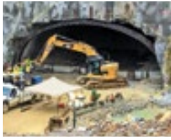
Drumanard Tunnel, Louisville, KY, USA
