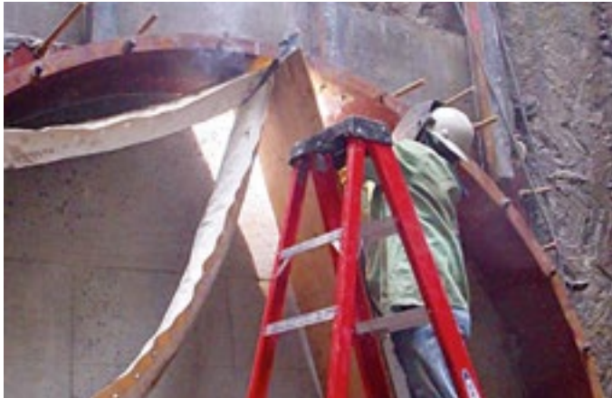
Welding of screws to the sealing holder Note: BULLFLEX® hoses must be protected against sparks and molten steel
