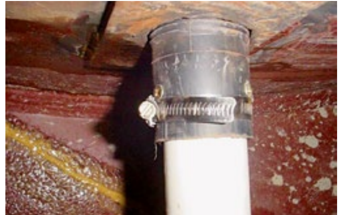
Stepwise grouting process of the sections (filling ports)
