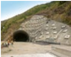
Loboguerrero Tunnel Chain, Valle del Cauca, Colombia
