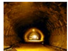
Thirra-Tunnel, Durrës, Kosovo – Albania
