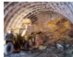
Upper Yeywa Hydropower Project, Myanmar
