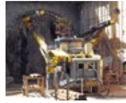
Tysons Corner, Dulles Corridor Metrorail Project, Vienna, VA, USA
