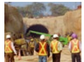
Rohtang Tunnel, Himachal Pradesh, India
