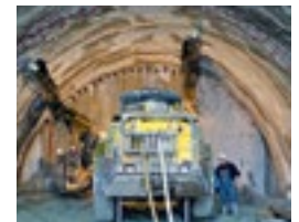
Omis Tunnel, National Road D8, Omis, Croatia
