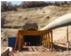
Alto Maipo Hydroelectric Power Plant, Maipo Valley, Chile
