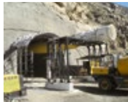
Cheves Hydroelectric Power Plant, Lima, Peru
