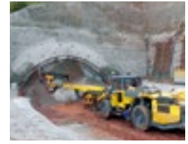
Hirschhagen Tunnel, Kassel – Herleshausen, Germany
