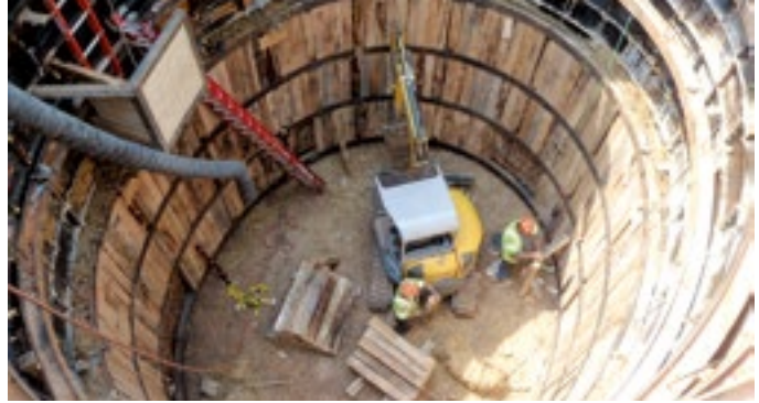
Shaft Rings and Breakout Structures
