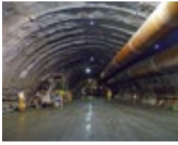
Caldecott Tunnel, Highway 24, Oakland - Orinda, CA, USA
