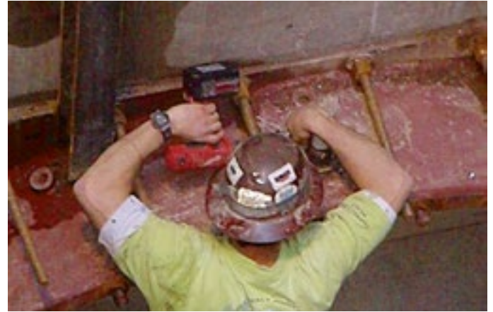
Fixation of filling pipes into the BULLFLEX® filling valves Note: to be able to ensure a proper grouting sequence, the filling pipes must be marked with different colors
